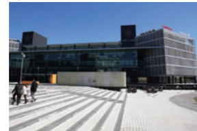
Spain PTA Malaga
